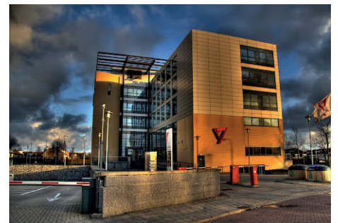
Seaway Heavy Lifting offices, Zoetermeer, The Netherlands. Source: Google Earth
